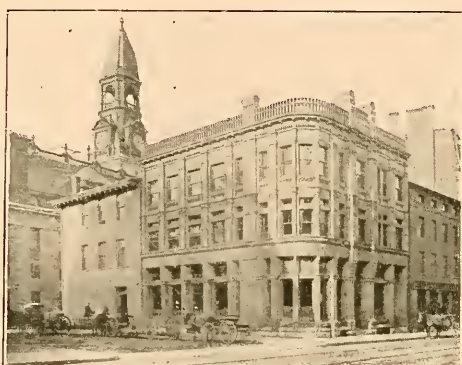
MASSASOIT BANK BUILDING, 33 BEDFORD ST.
